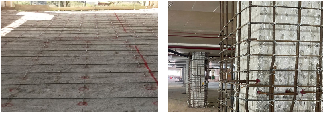
g) Slab shear-friction overlay
