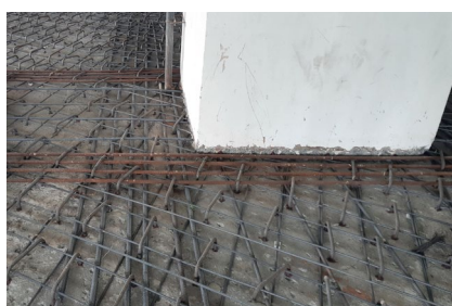
c) Slab strengthening
