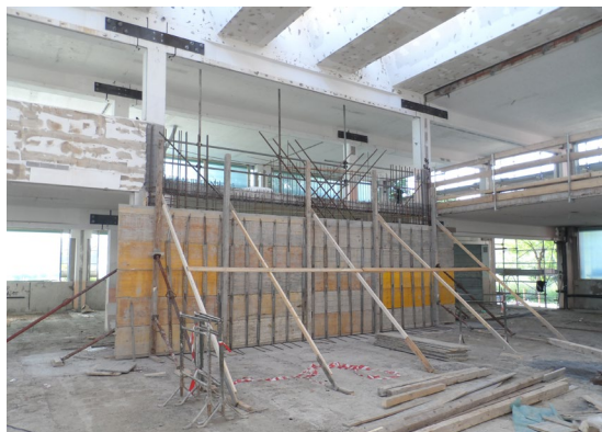
e) Shear wall addition
