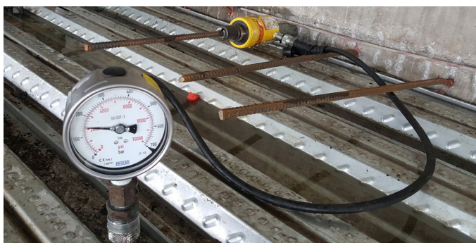
c) On-site inspection of post-installed rebars installation
