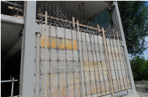
a) Corner walls
