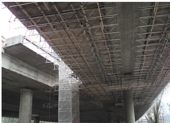
c) Increasing bridge girder thickness
