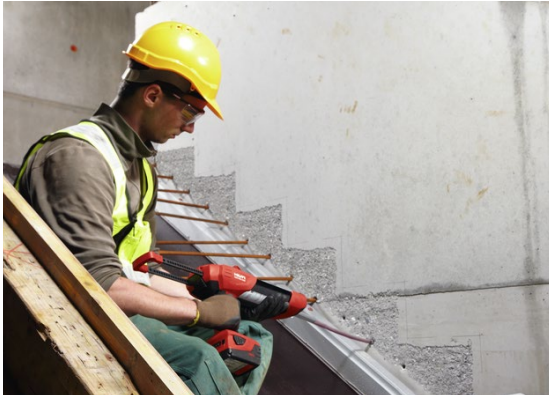
a) Stair-to-wall connection
