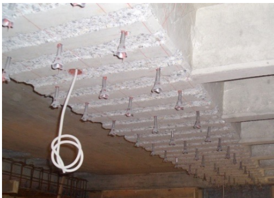
a) Increasing RC beam depth
