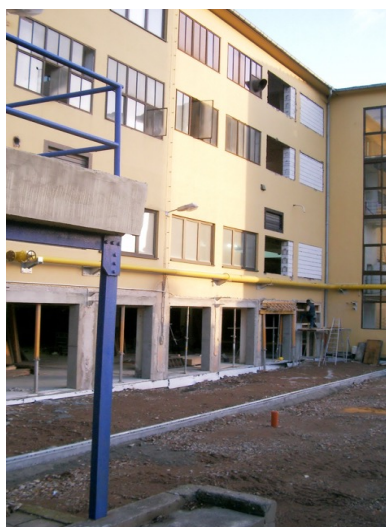
a) The 3 storey industrial building
