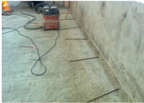
b) Connection of overlay to perimeteral walls
