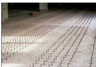
c) Slab strengthening with HCC-K shear connectors
