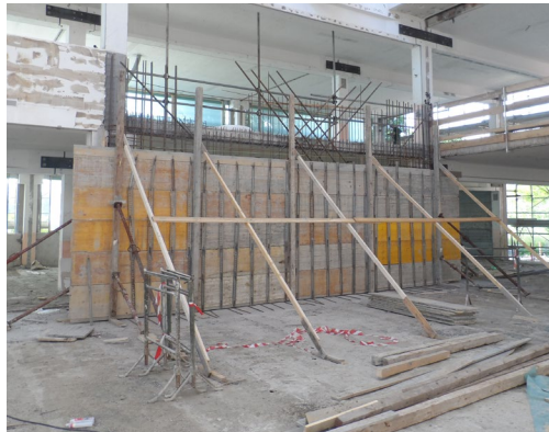
b) Interior walls
