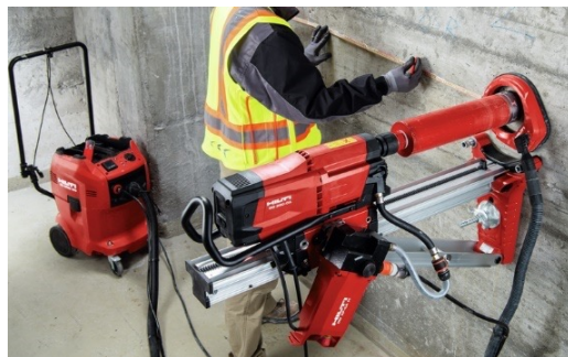
b) Diamond core drilling (Hilti DD 250 CA)
