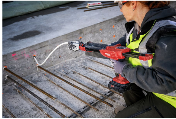
b) Extension hose for adhesive mortar injection
