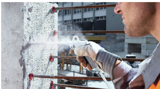
a) Air blow-out of dust from boreholes
