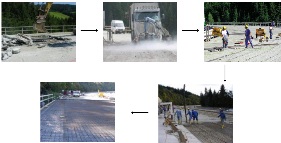
Fig. 9.18: Construction sequence of shear-friction overlay slab application (images in clockwise order)
