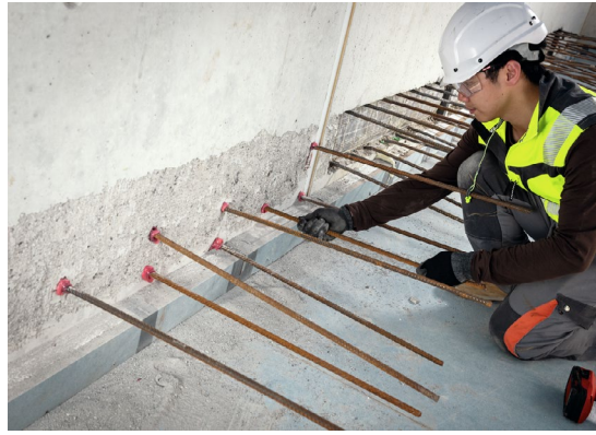
b) Slab-to-wall connection
