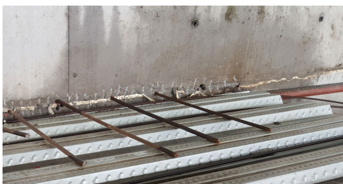
b) Post-installed rebars installation for slab to wall connection
