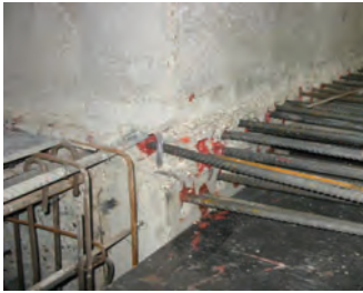
a. Slab-to-wall connection
