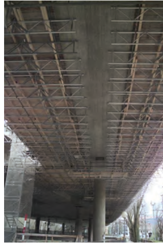
b. Bridge deck rehabilitation
