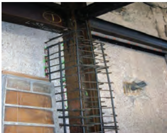
e. Steel column encasement extending from wall
