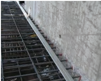
c. Slab-to-wall connection
