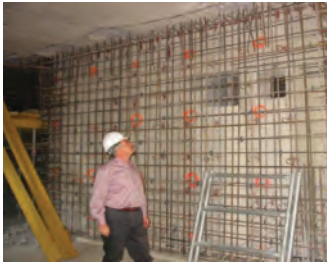
c. Onlay shotcrete wall
