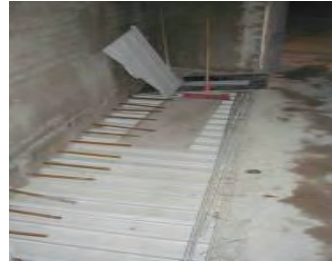
b. Slab-to-slab connection
