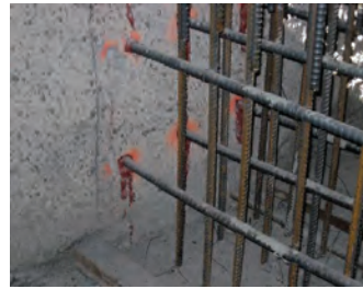
b. Wall-to-wall connection
