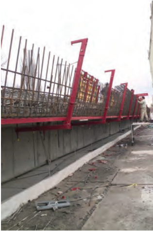
a. Bridge widening
