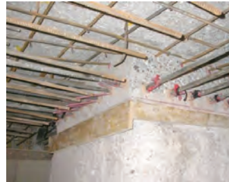
d. Slab-to-column connection strengthening
