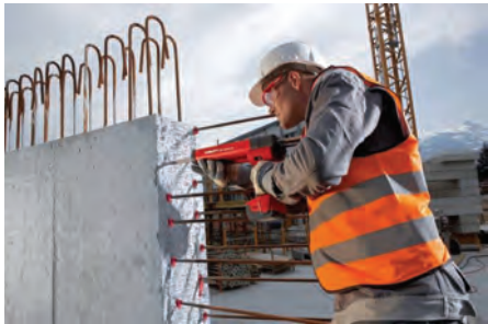
Figure 2– Injecting Hilti HIT adhesive in a drilled hole with Hilti dispenser HDM / HDE to simplify installation of post-installed reinforcing bars.
