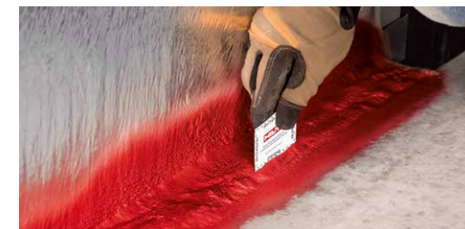
Hilti Firestop Spray: Enables fast and efficient sealing of wide joints, where maximum movement is required – e.g. curtain wall joints or openings between walls and ceilings.
