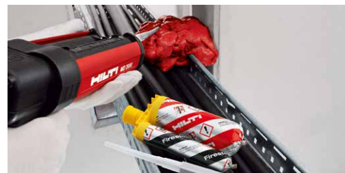
Hilti Firestop Flexible Foam: A reliable firestop seal for all types of cable penetrations, offering quick installation, easy maintenance and retrofitting of cables.
